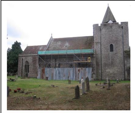
The Kent peg tiles on the North side of Leeds church roof had deteriorated with age and the area over the North aisle, which has a less steep slope, and is subject to moss growth, was particularly bad and needed completely renewing. Other areas of the roof needed limited repairs. We are pleased to report that these serious deteriorations have now been repaired and the Friends contributed £6,000 this year towards the cost. Picture opposite shows the work underway.
